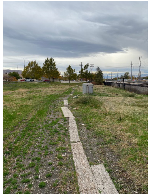
Figure 27: The informal path covered in plywood near the Woods Cross FrontRunner station.
